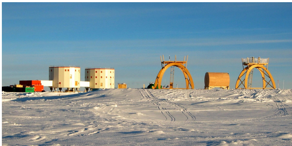
Figure 1. Starting in 2005 the two 3-storey towers of the Concordia station at Dome C will accommodate a small population of 16 winter-over scientists and technical staff. The 5-m high wooden Concordiastro platform, on the right side of this image, supports the site testing telescopes.
